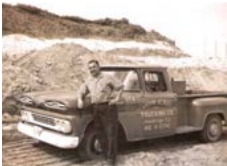
John Almasi Sr., founder of Almasi construction, stands with one of the original trucks of the Almasi Trucking fleet.
