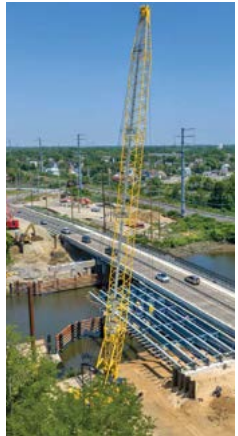
Reconstruction of the Route 130 bridge over Big Timber Creek.
