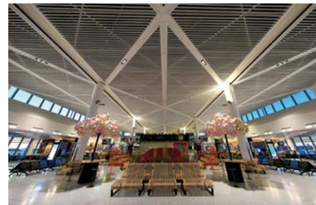
An inside view of the finished Terminal A
