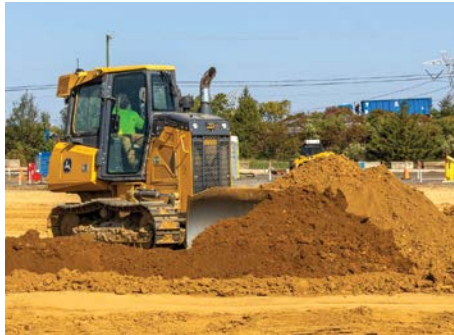
Dominic Serpineto practices moving piles of dirt.
