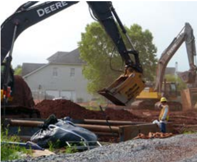
Pipeline passes beneath neighborhood roads.
