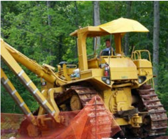
Sidebooms support the pipeline while welding takes place below.
