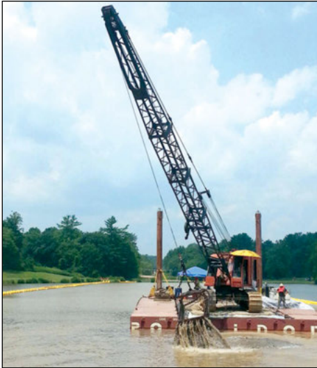
A 98 Link-Belt crane digging ditch across McCormack Lake.
