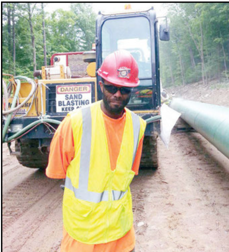
Tyson Hill, Local 825 apprentice, runs a sandblaster on the coating crew.
