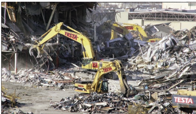
Dismantling the old General Motors plant in Linden, three years ago.
