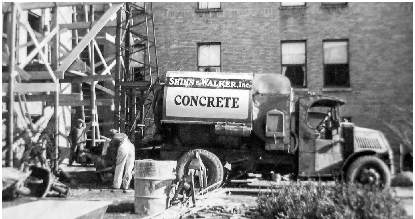
Early 1940s: One of Shinn & Walker's ready-mixed concrete trucks utilizing Edward Shinn's patented truck-mounted hoists.
