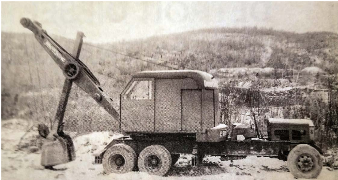
One of United Crane & Shovel's early vintage truck-mounted Browning shovels on site in 1941 at the Picatinny Arsenal.
