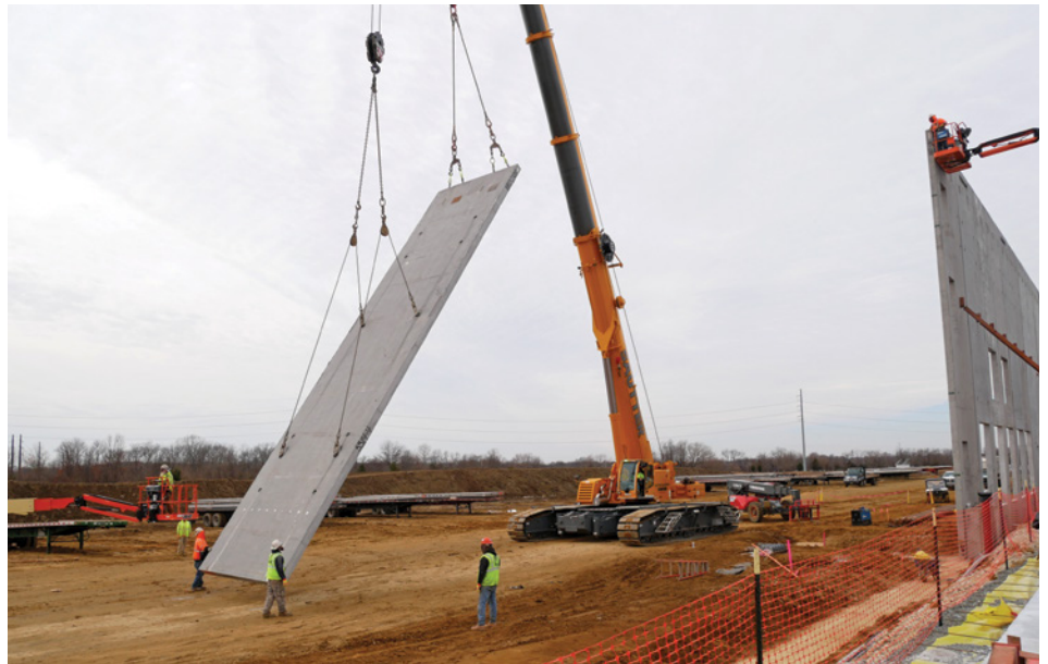
MRP PROJECT – The Amazon Warehouse being constructed in West Deptford Township by Petillo Construction Inc. was assisted by a Market Recovery Program grant from ELEC.]
